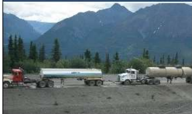
Asphalt Pavement In-place Recycling Technologies (APIPRT)
