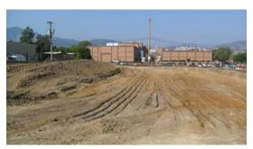
In 2006, Englewood based, Ground Engineering Consultants completed its study of subgrade conditions and determined that "materials encountered in our test holes consist of fine to coarse-grained sand in the upper 5 feet. According to the National Asphalt Pavement Association (IS-131), these materials appear to be suitable for a porous pavement section."
